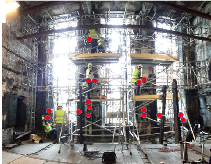
Figure 1: overview of the damaged sandstone piers in the Library of the Mackintosh Building. View is facing west, and the red dots indicate the location of analysis points, including of taken-down stone (i.e. not an in-situ measurement) for the highest located point.
